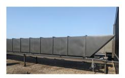
Pro-R Double Wall is a preinsulated duct solution suitable for outdoor and indoor applications.
